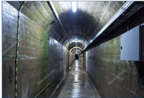
Construction of dams
