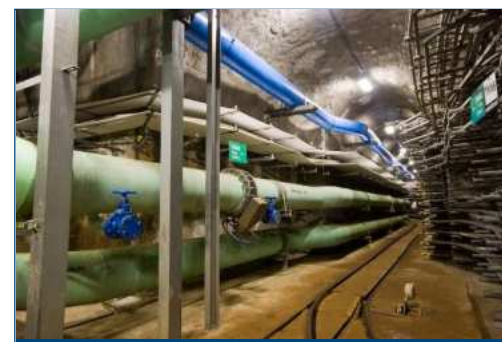
Extending / renovation of utility tunnels
