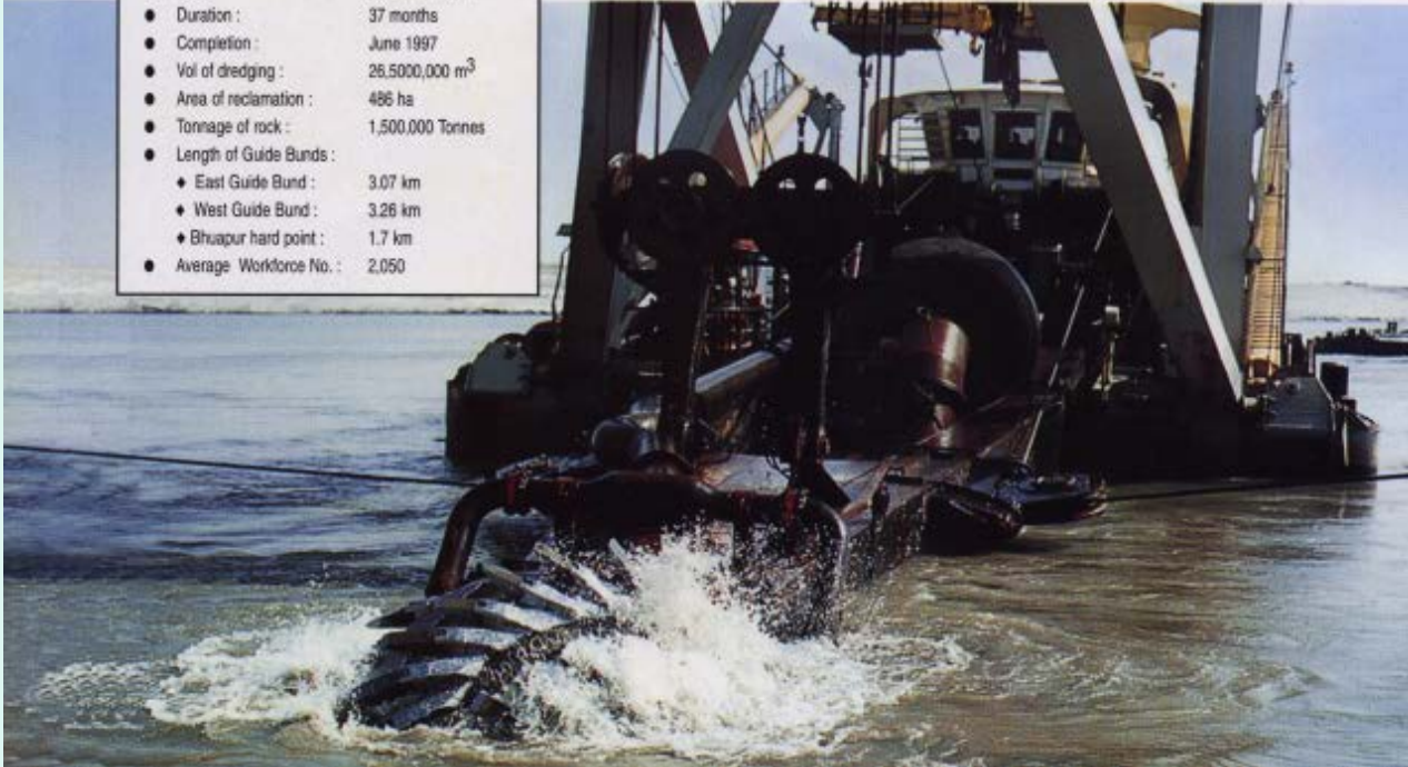
Dredger at Work
